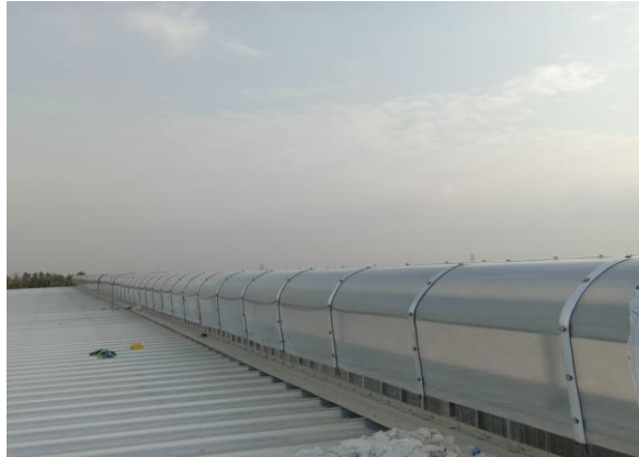
Roof monitor at SVS Warehouse, Bangalore
