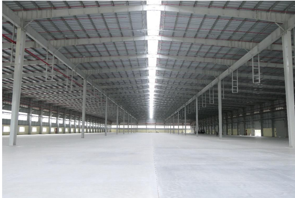
Inside view of Roof monitor at SVS warehouse, Bangalore The building is flooded with Diffused Natural Light
