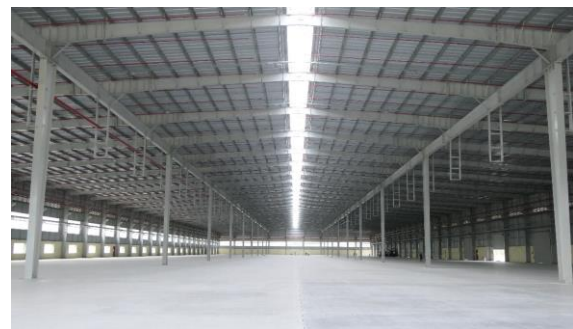
Roof monitor at SVS warehouse, Bengaluru
